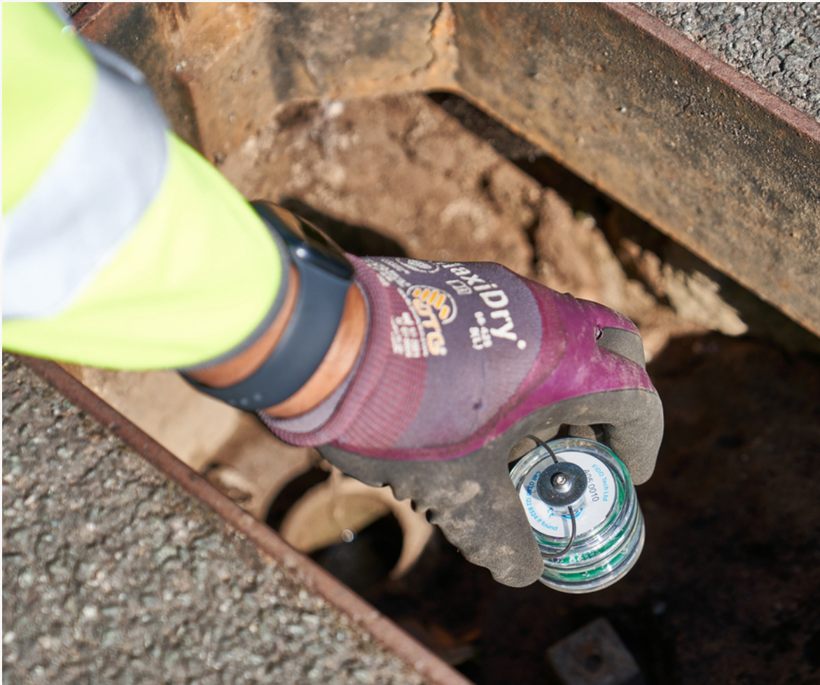
Placement of an acoustic sensor in water pipeline to detect leaks. | Image courtesy of FIDO Tech.
